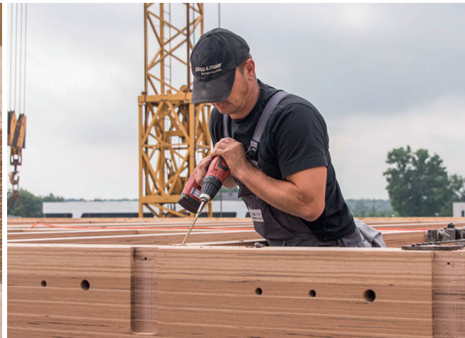
Connection between post and beam
