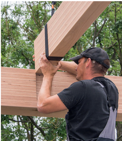
Connection between girder and auxiliary beam
