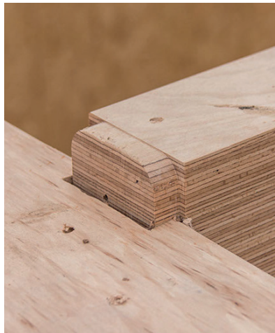
Connection between girder and auxiliary beam
