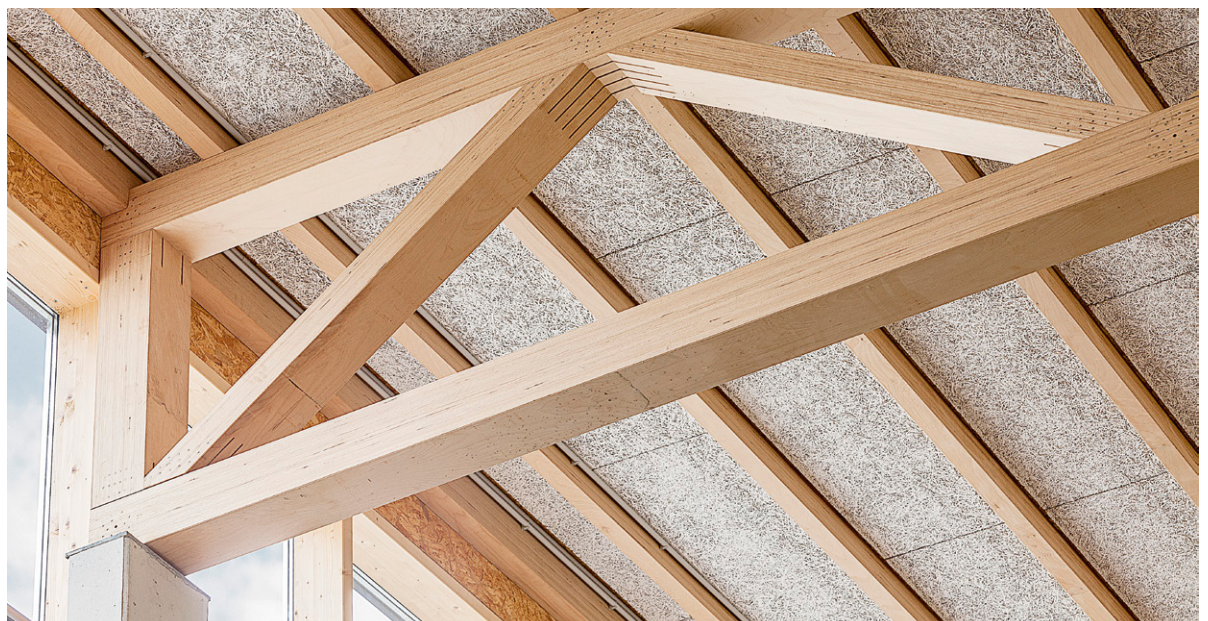
BauBuche truss with BSB connections, i+R Holzbau
