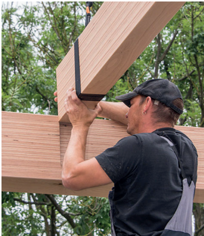
Connection between girder and auxiliary beam
