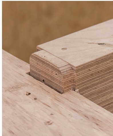
Connection between girder and auxiliary beam
