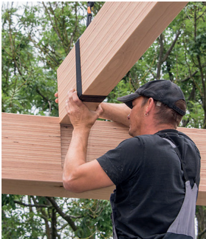
Connection between girder and auxiliary beam
