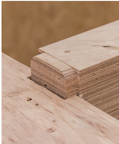
Connection between girder and auxiliary beam
