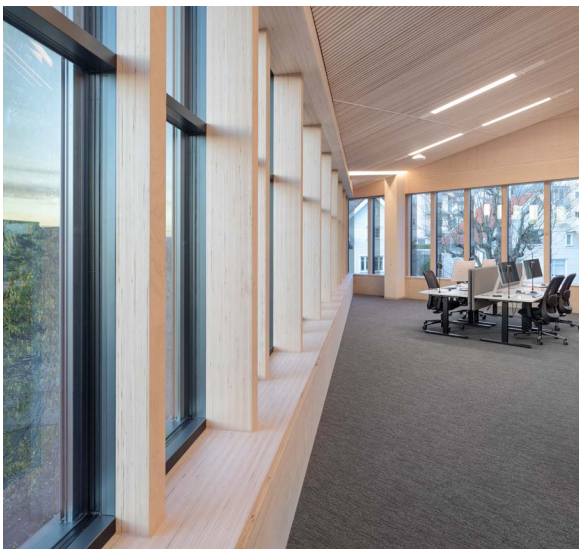
The new office block of SR Bank in Stavanger (Norway) is built primarily in timber BauBuche was used for the posts at ground floor level and for many other building elements. Architects Helen & Hard Architects in cooperation with SAAHA architects Timber construction Moelven
