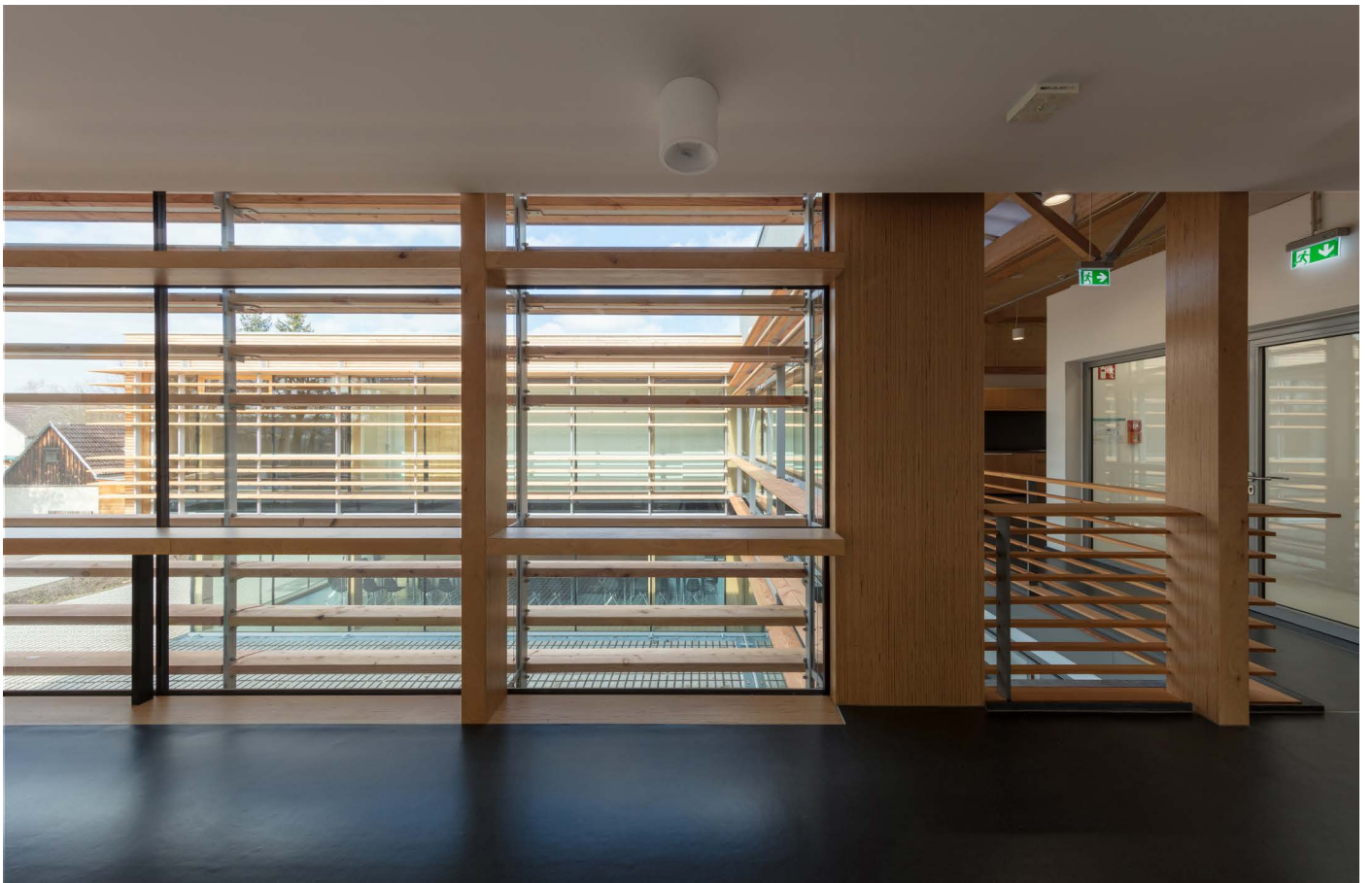
Skeleton frame made in BauBuche, Jena Forestry Office, Stadtroda Locally sourced timber was the material of choice for the construction of the local forestry office. Architects cornelsen + seelinger architekten BDA Timber construction Grossmann Bau GmbH & Co. KG Supporting structure planning merz kley partner ZT GmbH
