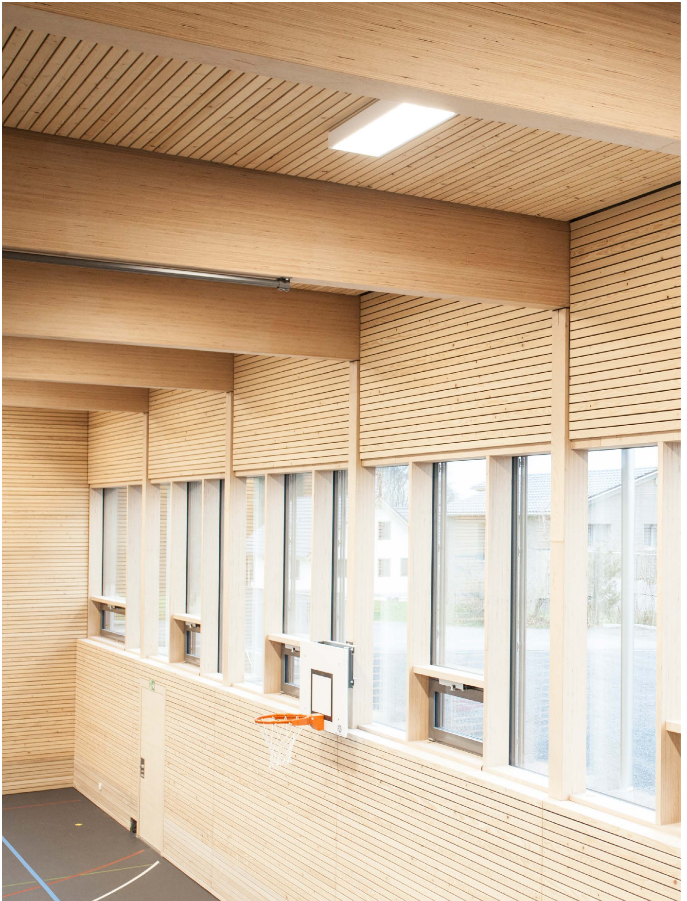
New gym hall, Islisberg The girders span 12.60 m but measure only 90 cm in height and 20 cm in width. Architects Langenegger Architekten AG, Muri Structural design Makiol Wiederkehr AG, Beinwil am See Timber construction Max Vogelsang AG, Wohlen
